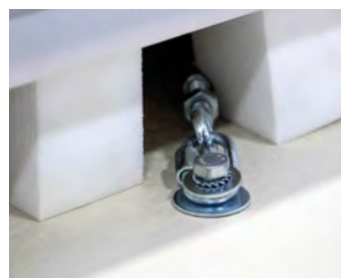
Detail of the anti-rotation kit.
