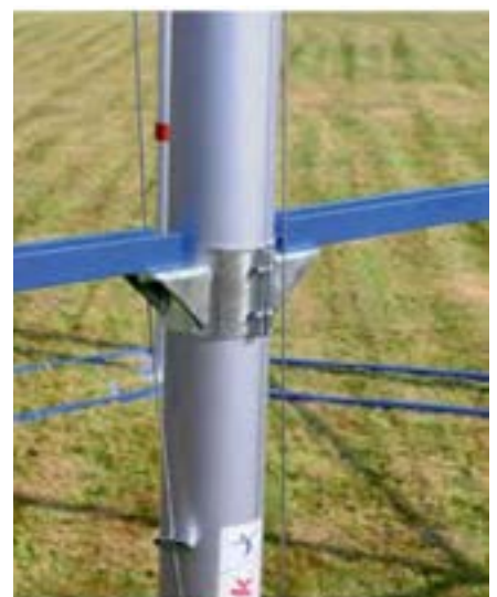
upper steel powder painted connectors bond cage pillars together
