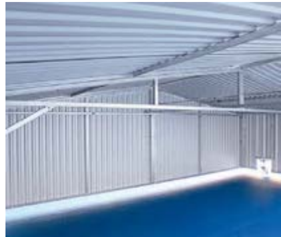
supporting construction made of hot galvanized steel, aluminium sheet roof and sides
