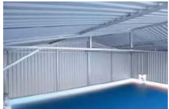
supporting construction made of hot galvanized steel, aluminium-zinc sheet roof and sides
